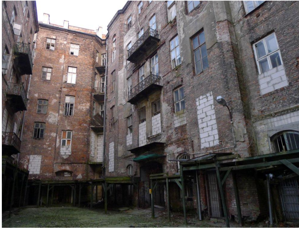
Próżna 9 – The courtyard of the neglected building. March 2014
