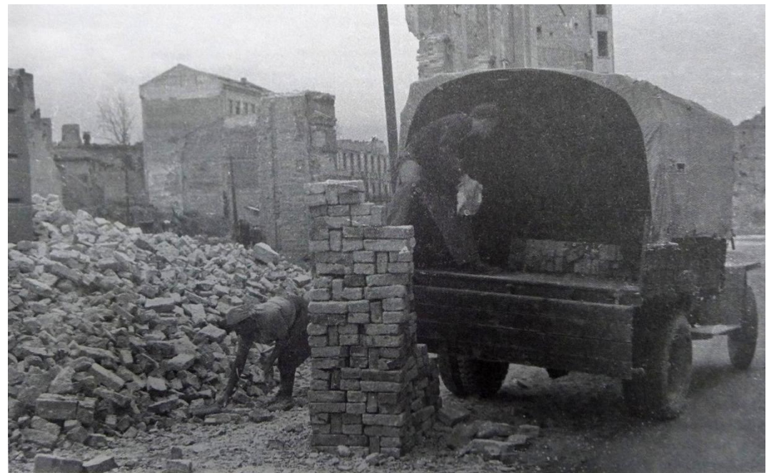
Reusing building material in Nalewki St., May 1947
