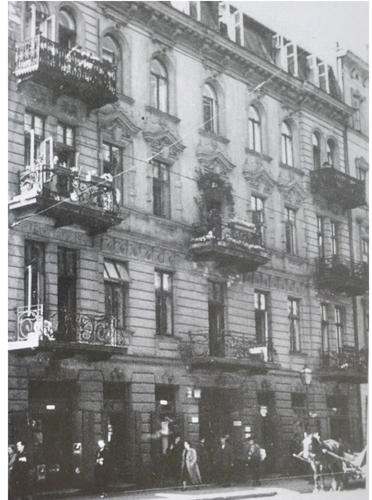
Apartment building in Nowolipie 66, 1938
