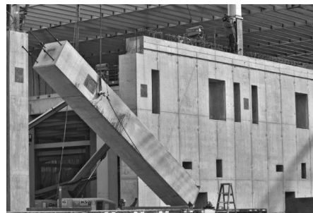
“2D Tree” columns are easier to be pre-fabricated and assembled on site
