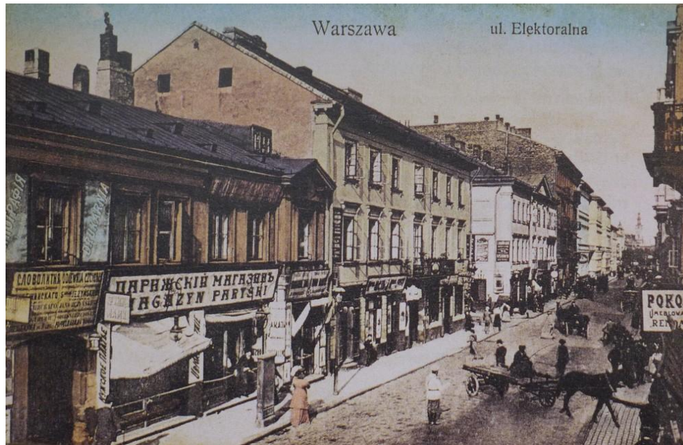
Elektoralna St. Before World War I. Continuous street facades were evolved in the 18th century.
